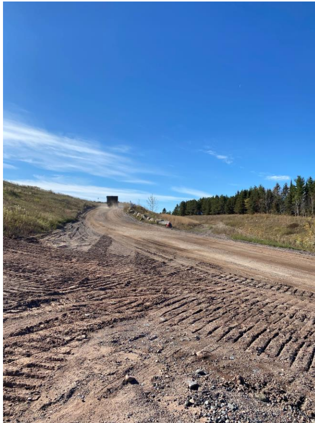
Location 3 – Looking West, Phase 2 Northern Waste Slope & Berm
