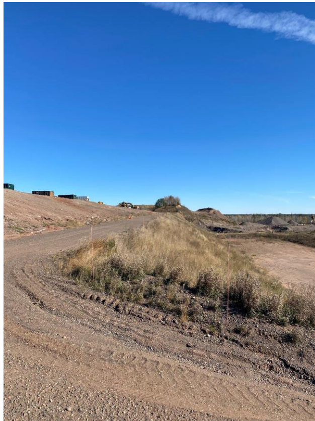
Location 5 – Looking East, Phase 5 Southern Berm
