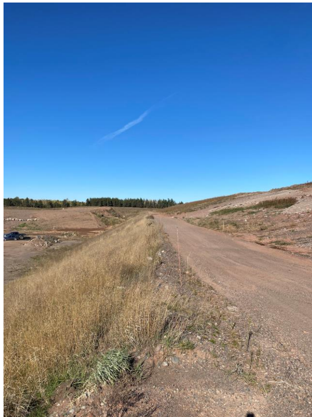
Location 5 – Looking North, Phase 2, 3, 5 Western Berm
