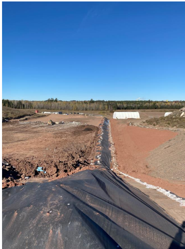
Location 10 – Looking North, Cell 7 Eastern Berm
