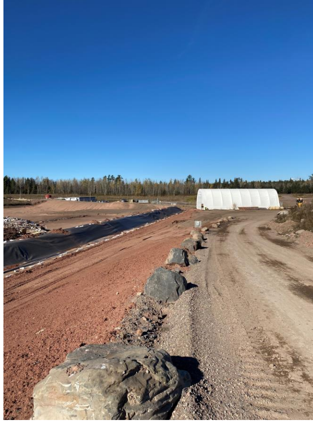
Location 11 – Looking North, Cell 7 Eastern Berm
