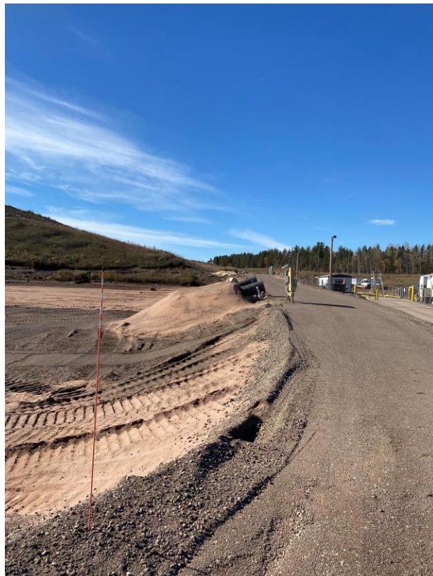
Location 1 – Looking West, Phase 7A Northern Berm
