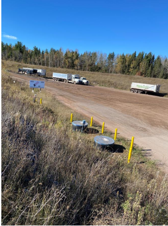
Location 3 – Looking North Phase 1
