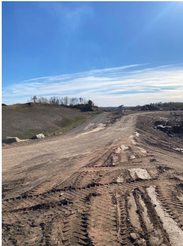
Location 9 – Looking South, Phase 4 East Road
