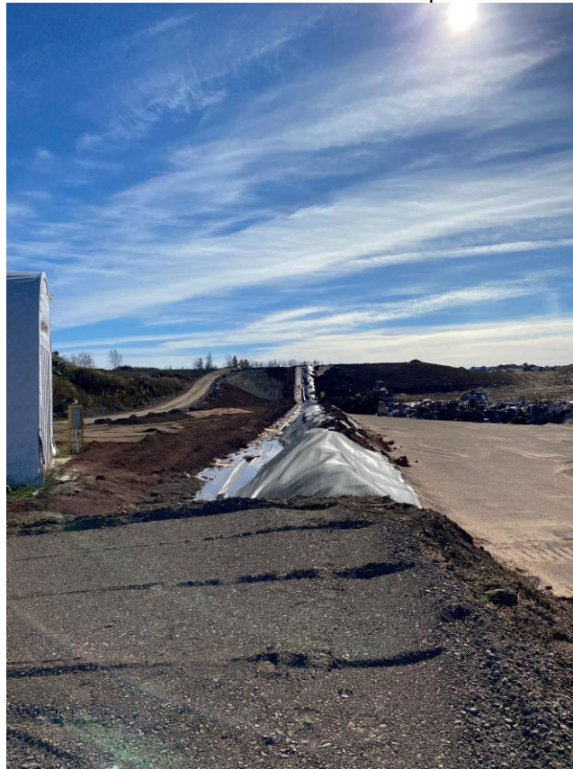
Location 1 – Looking South, Phase 7A Eastern Berm
