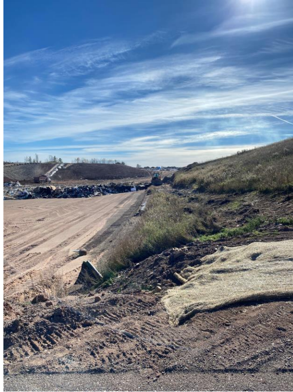
Location 2 – Looking South, Phase 1 Eastern Berm
