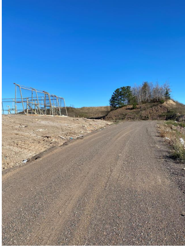
Location 6 – Looking East, Phase 6 Southern Road
