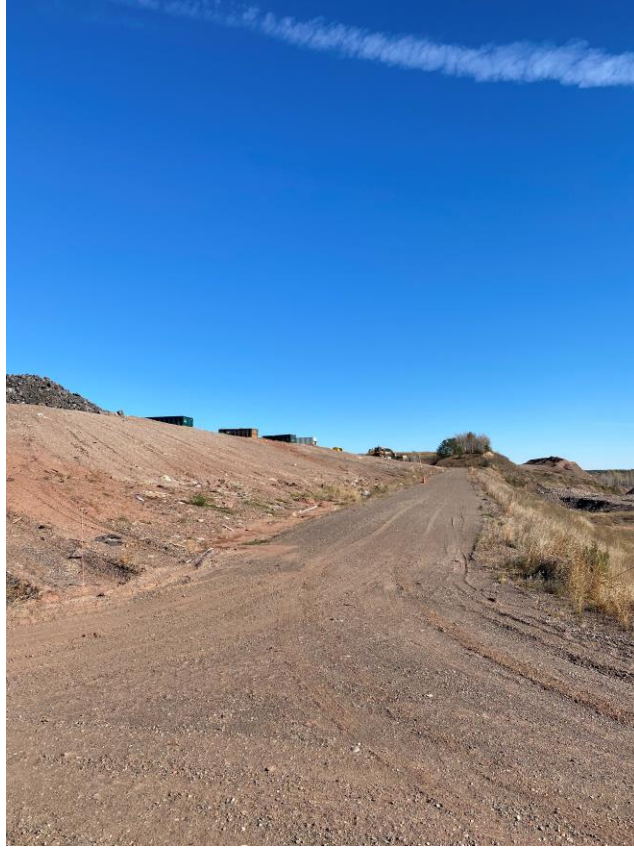
Location 5 – Looking East, Phase 5 Southern Road
