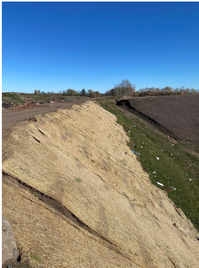
Location 9 – Looking East, Cell 7 Berm
