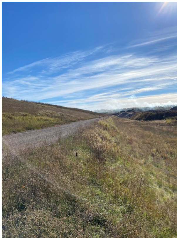
Location 4 – Looking South, Phase 2 Western Berm
