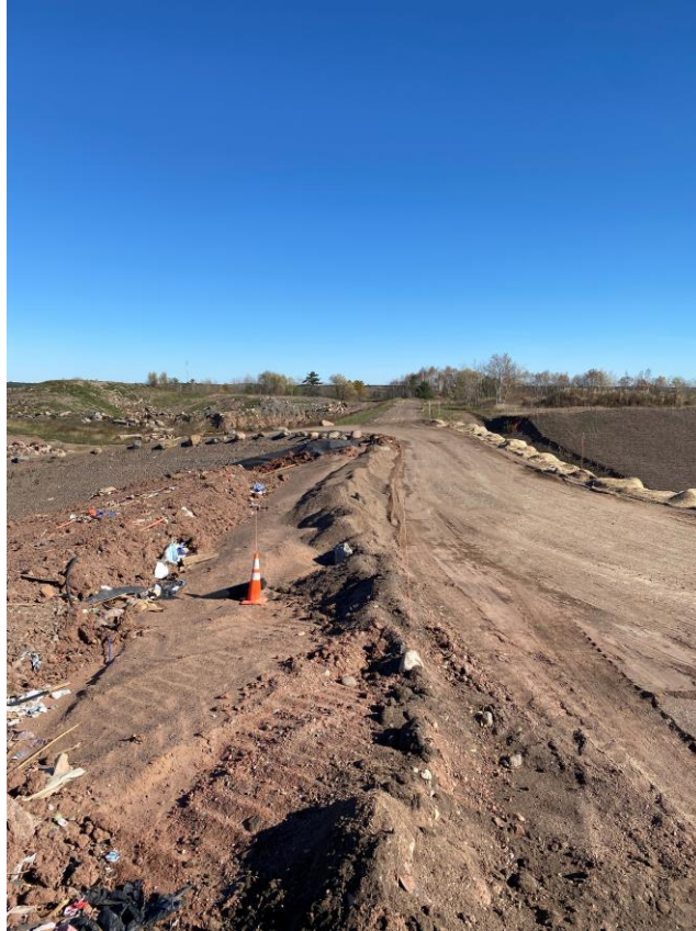
Location 9 – Looking East, Cell 7 Southern Anchor Trench
