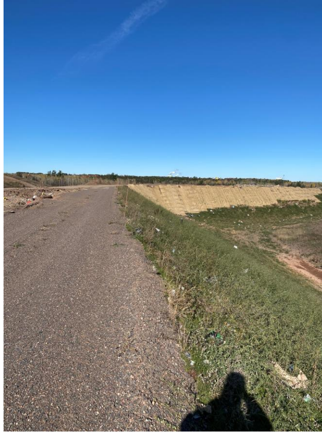
Location 8 – Looking North Phase 4 Berm
