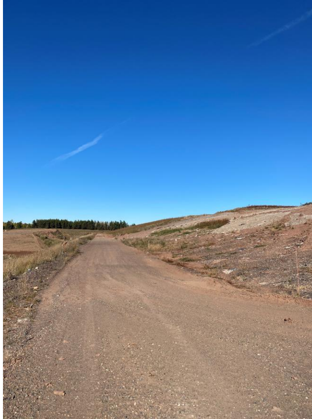
Location 5 – Looking North, Phase 2, 3, 5 Road & Berm
