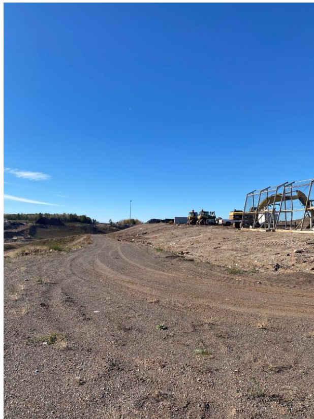
Location 7 – Looking West, Phase 6
